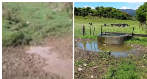
Stock and vehicle crossing that needs a culvert
