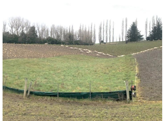
Grassy swale protecting CSA
