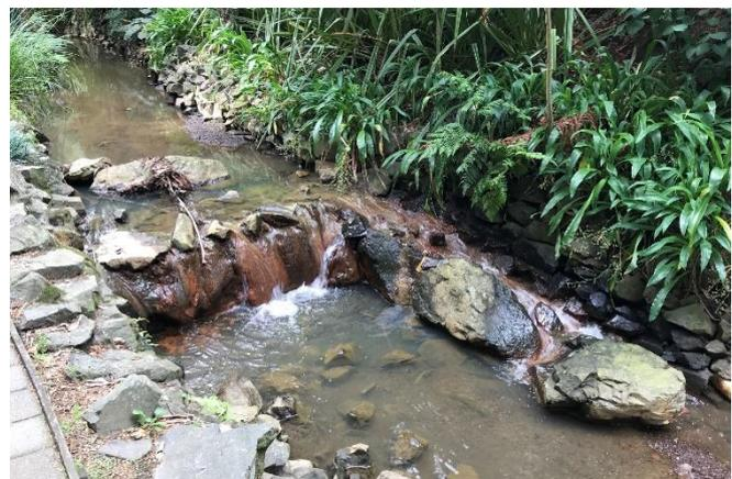
**Figure 2:** After installation of a concrete rock ramp to provide passage for swimming fish species, March 2016. Photo: NIWA
