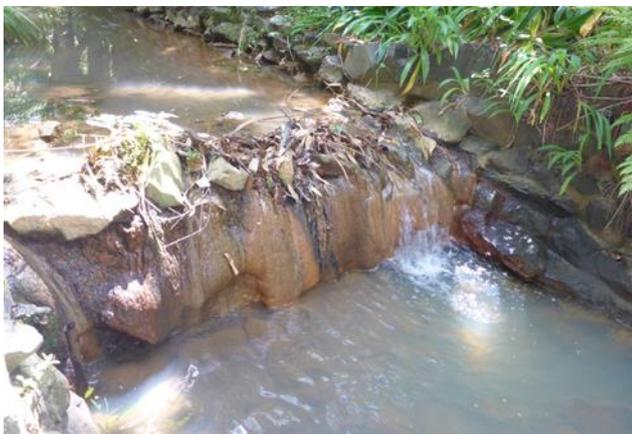
**Figure 1:** One of four weirs on Gibbons Creek that impeded passage for weak swimming fish, December 2015.
